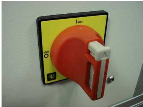
Part #170 (Emergency Switch)
